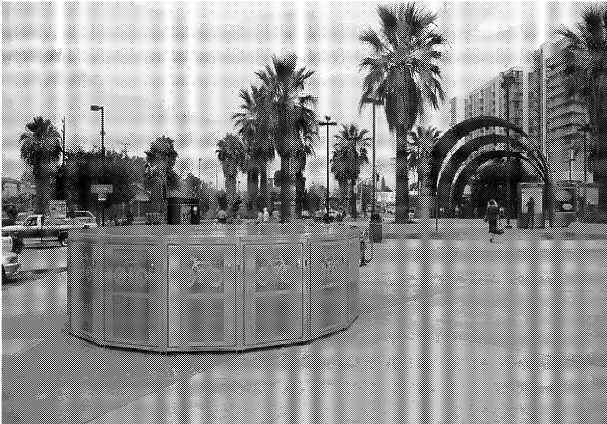
Bicycle Lockers at North Hollywood Red Line Station
