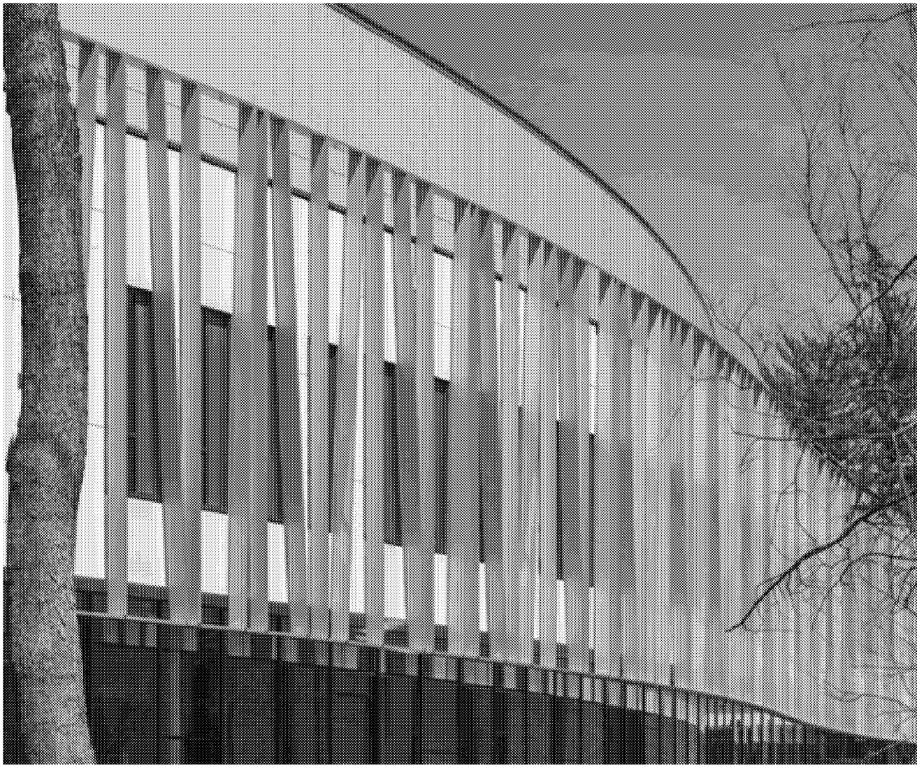
Southeast facade; Ornilux and solar screen fins (©Richard Barnes)
