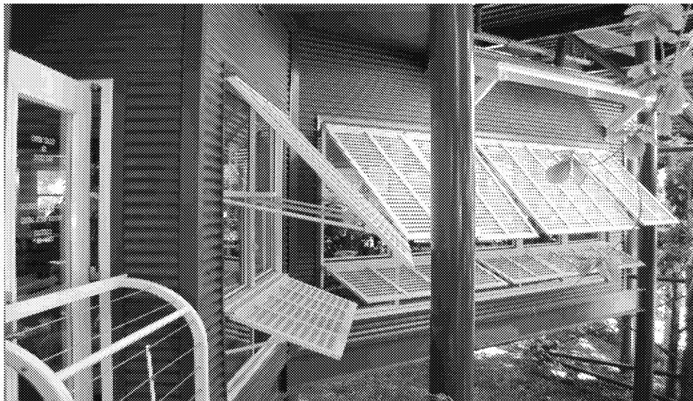
Shutters overhang windows at a facility at the San Diego Zoo. Photo by Christine Sheppard, ABC
