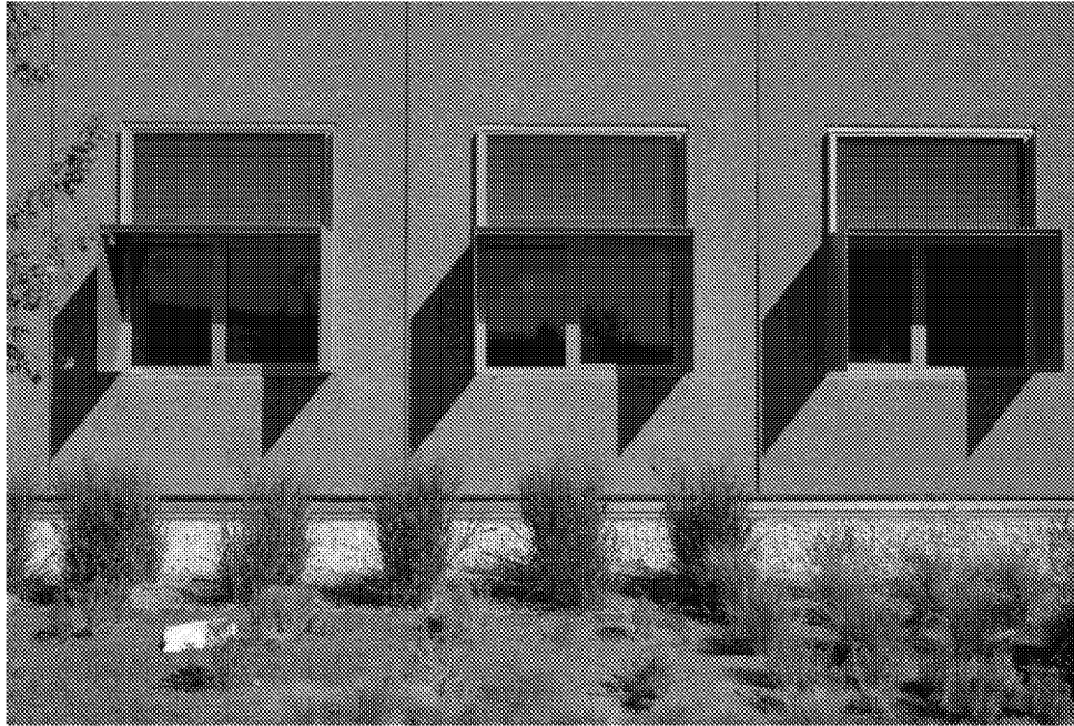
Shading was applied around the windows on the exterior of the Research Support Facility (RSF) at the National Renewable Energy Laboratory (NREL) to reduce glare and overheating of the building interior. These windows are also bird friendly. Photo by Dennis Schroeder, NREL 19798
