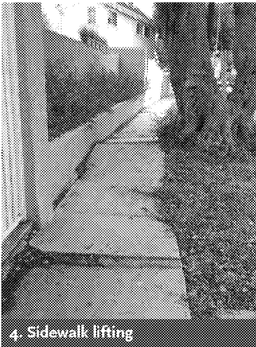
1. Sidewalk lifting
