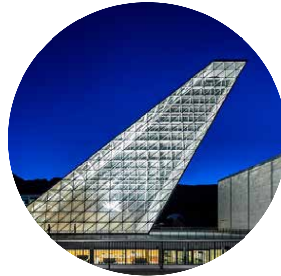
Lighting Highlighting Architectural Elements
