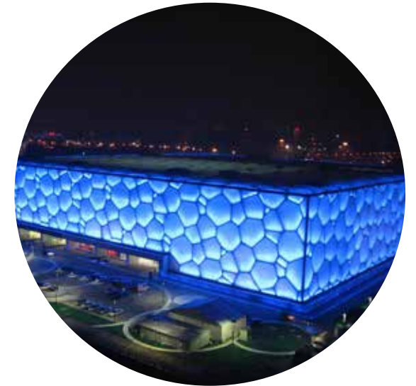
Exterior Facade Lighting
