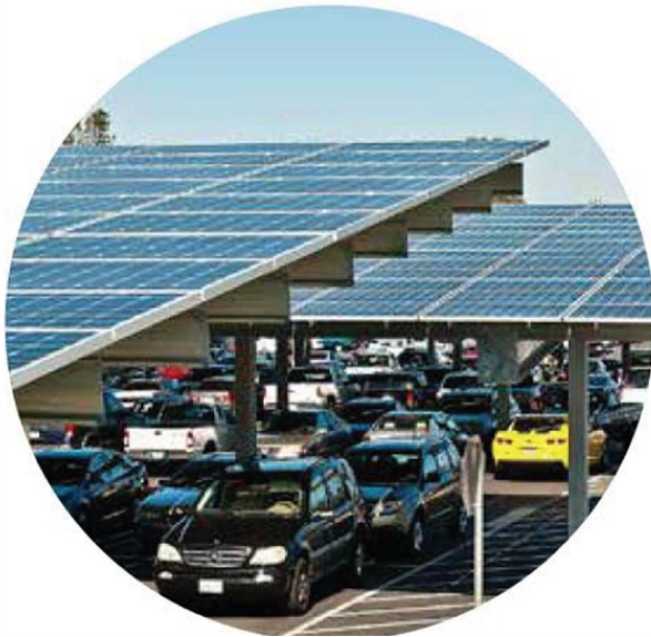
Roof Structure Solar Panels
