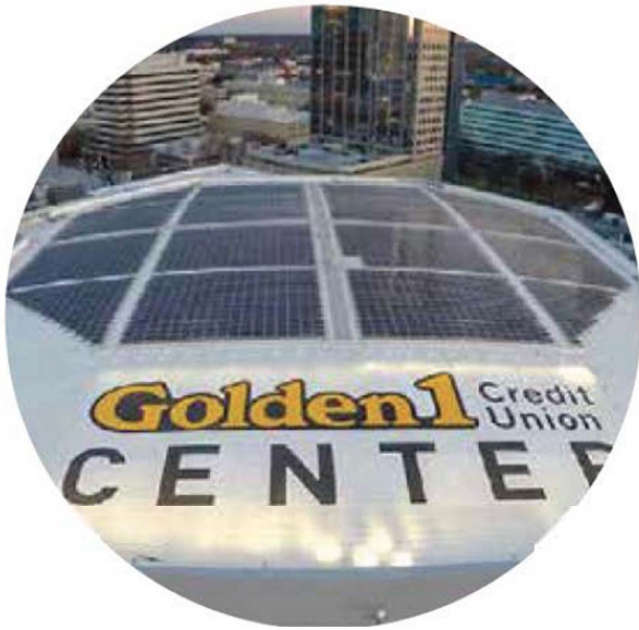
Integrated Roof Top Solar Panels
