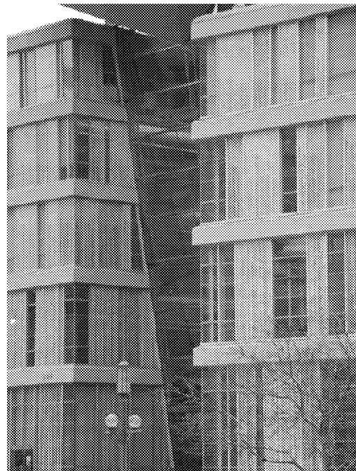
Minnesota Eco-Cafe Building Guidelines
