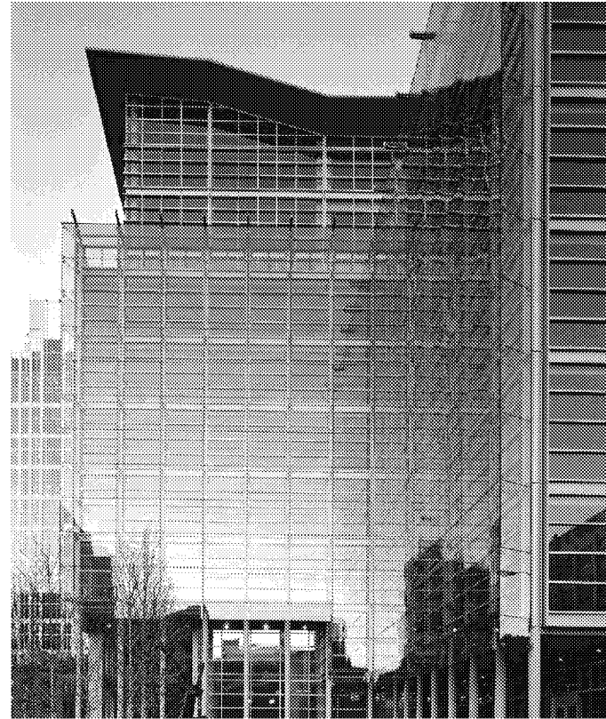
TOP: SoMa's Foundry Square presents a full façade of highly reflective glass. While all glass can be reflective, glass manufacturers label glass with standards "reflectivity" ratings.
