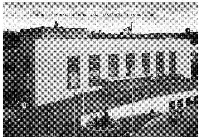
ABOVE: Many historic buildings such as the old Transbay Terminal present a solid appearance.
