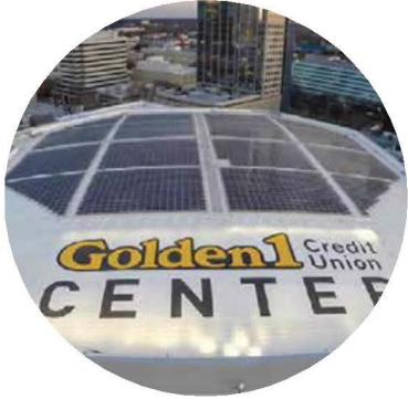
Integrated Rooftop Solar Panels
