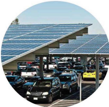
Roof Structure Solar Panels
