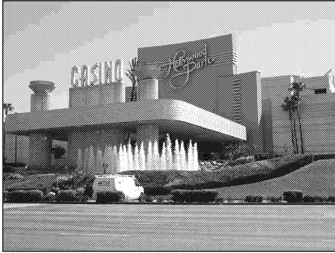
View 4: View of Hollywood Park Casino from the on-site parking lot.
