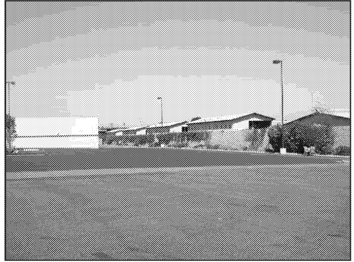
View 14: View of Hollywood Park Stables and adjacent commercial shopping center.
