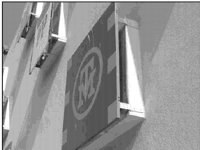
Photograph 3: Detail of wood vent covers decorated with owners' silks, December 2006.
