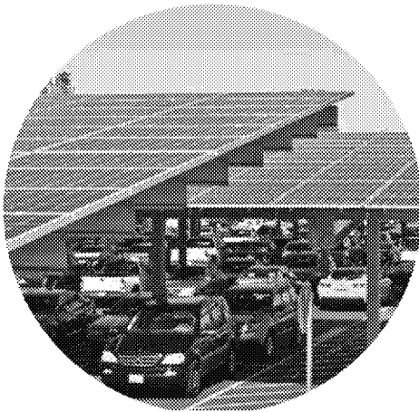
Roof Structure Solar Panels
