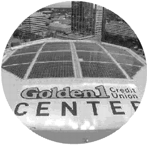
Integrated Rooftop Solar Panels
