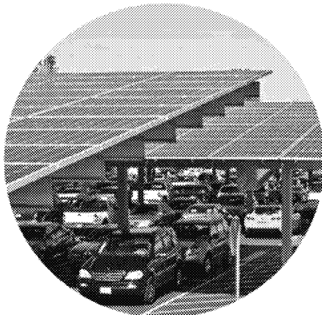
Roof Structure Solar Panels
