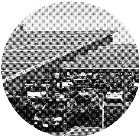
Roof Structure Solar Panels
