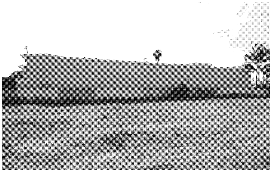
East (side) façade, view facing west. ESA, 2018.
