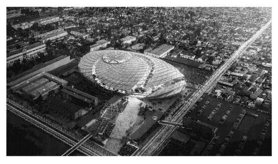
An aerial view rendering of the Clippers' proposed 18,500-seat arena in Inglewood. The oval design has a unique exterior of diamond-shaped metal panels inspired by the concept of a basketball swishing through a net. File photo
