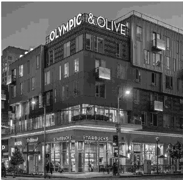
Olympic & Olive, Los Angeles, CA
