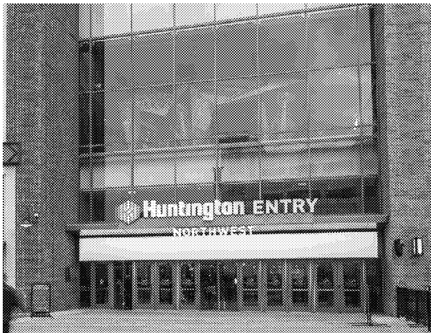
Northwest Entry, Little Caesars Arena, Detroit, MI
