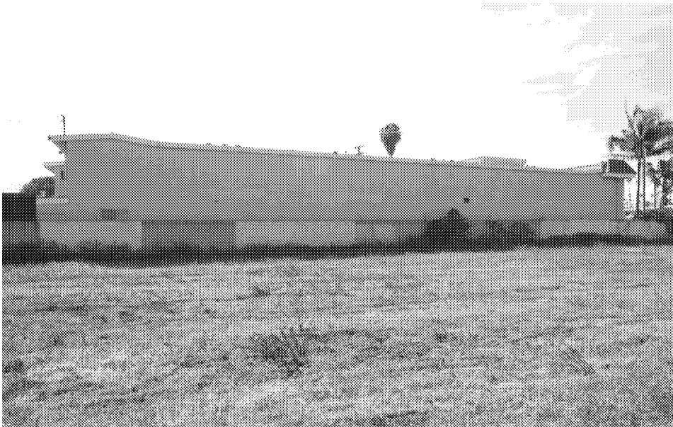
Figure 24 East (side) façade, view facing west
