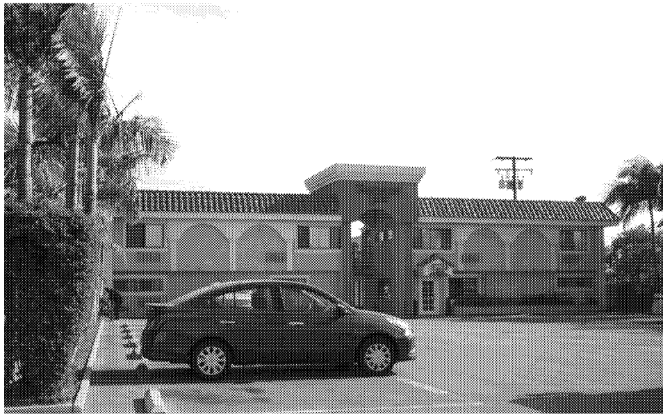
Figure 22 North (front) façade, view facing south
