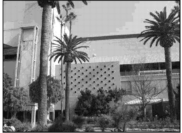
Photograph 5: Main building, Turf Club and Clubhouse wing. December 2006.
