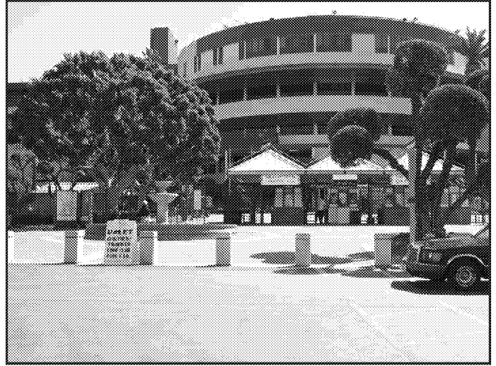
View 2: View of the main entrance of Hollywood Park Racetrack from Hardy Street facing east.
