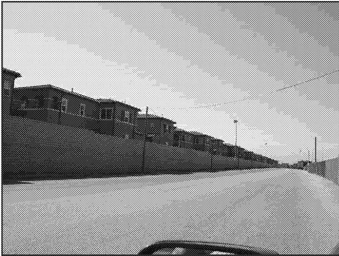
View 36: View from the intersection of 90th Street and Carlton Way looking south. The Project Site is located south and adjacent residential uses are located to the east (left).
