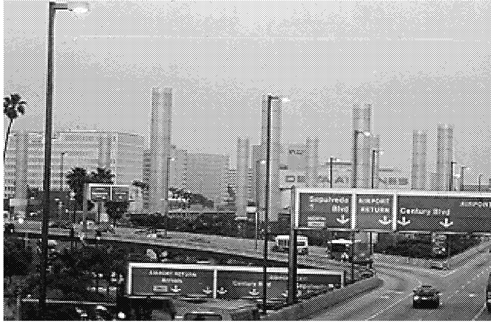
Day time View of LAX Gateway Circle Pylons
