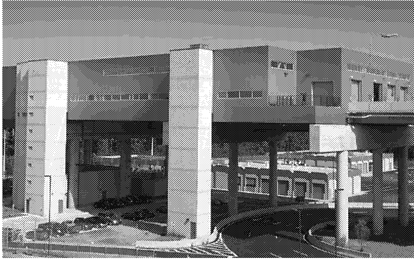
ATL ConRAC (Atlanta International Airport) MSF (above roadways, and in between ConRAC garages)
