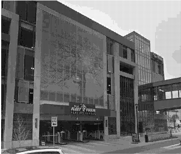
Mills Fleet Farm Parking Garage, Minneapolis, MN
