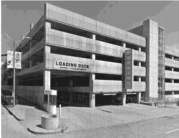
Loading Dock, Enterprise Center, St. Louis, MO
