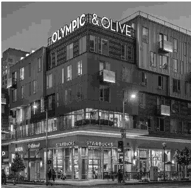
Olympic & Olive, Los Angeles, CA
