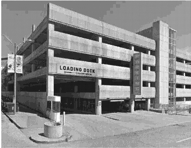
Loading Dock, Enterprise Center, St. Louis, MO
