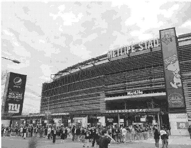
Digital Pylons at Entrance Gates, Met Life Stadium, NJ
