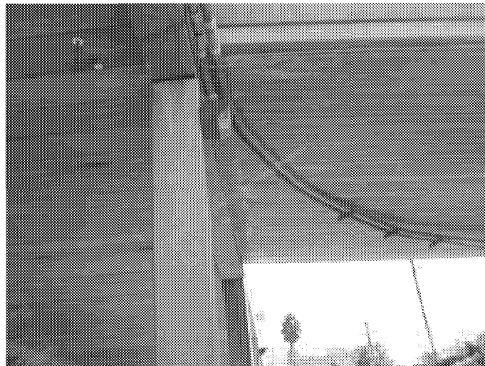
Figure 5.5 Bridge Connection to the Building
