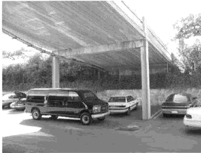
Figure 5.4 Parking Level Bridge
