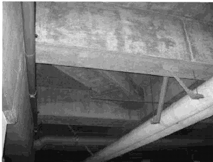
Figure 5.5 Girders supporting Shear Wall Above
