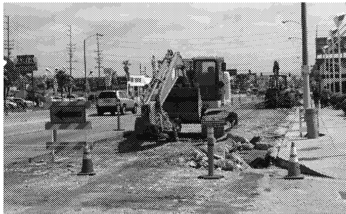
Figure 4- 6: Reconstruction of La Brea Avenue (6/2013)
