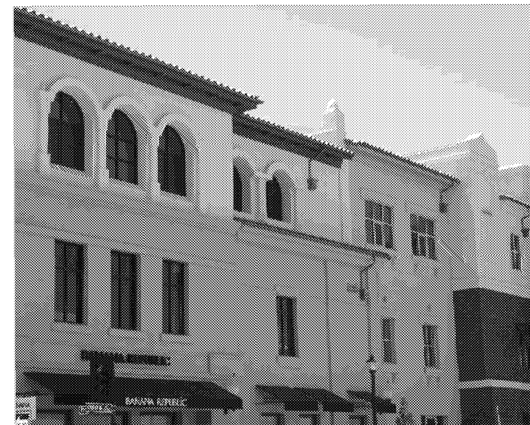
Example - Varying Window Designs, Roof Treatments, Material Changes and Wall Plane Offsets Generate Visual Interest and Reduce the Scale of this Large Scale Building
