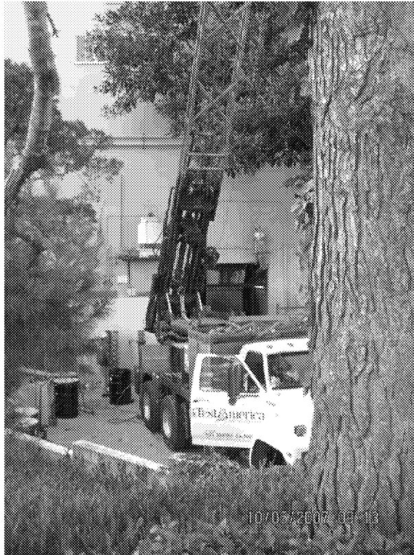
Photo 5: Drilling of borehole for SVE-1 outside the Former Dry Cleaning Area, looking south, 5 October 2007
