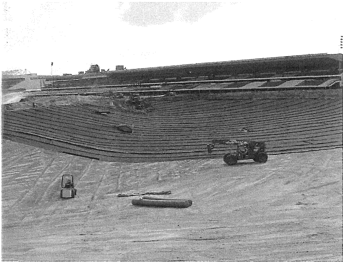
Placement of the geotextile fabric over geosynthetic liner and 6 inch soil cover on 9/7/00.
