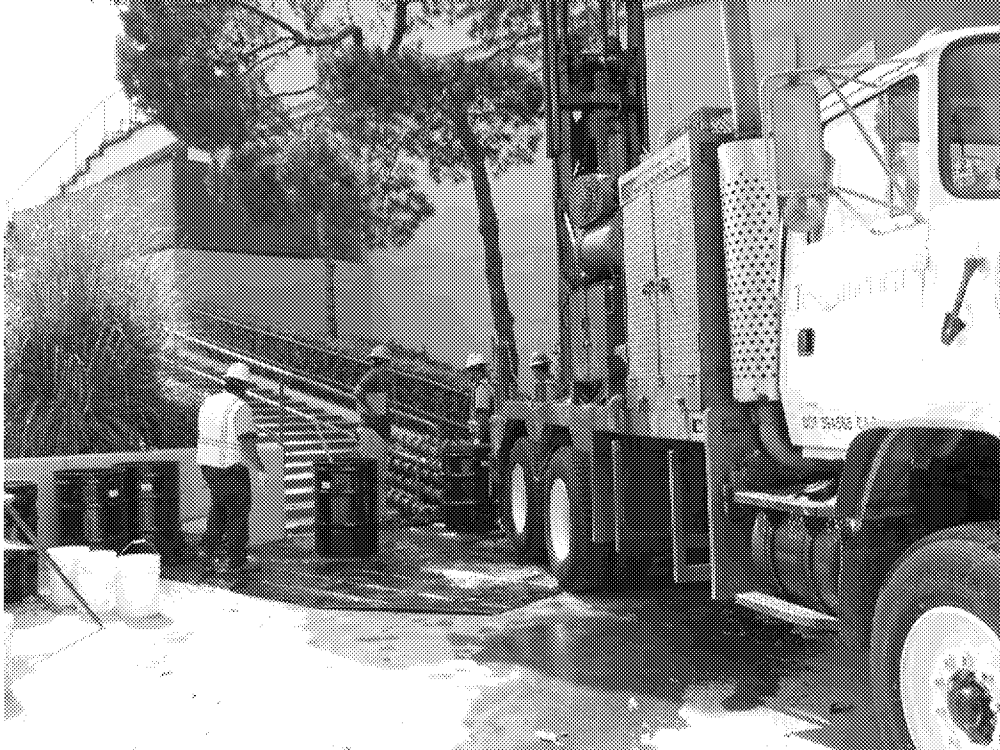
Photo 3: Drilling of borehole PS-GW-1 outside the Former Dry Cleaning Area, looking southeast, 27 June 2005
