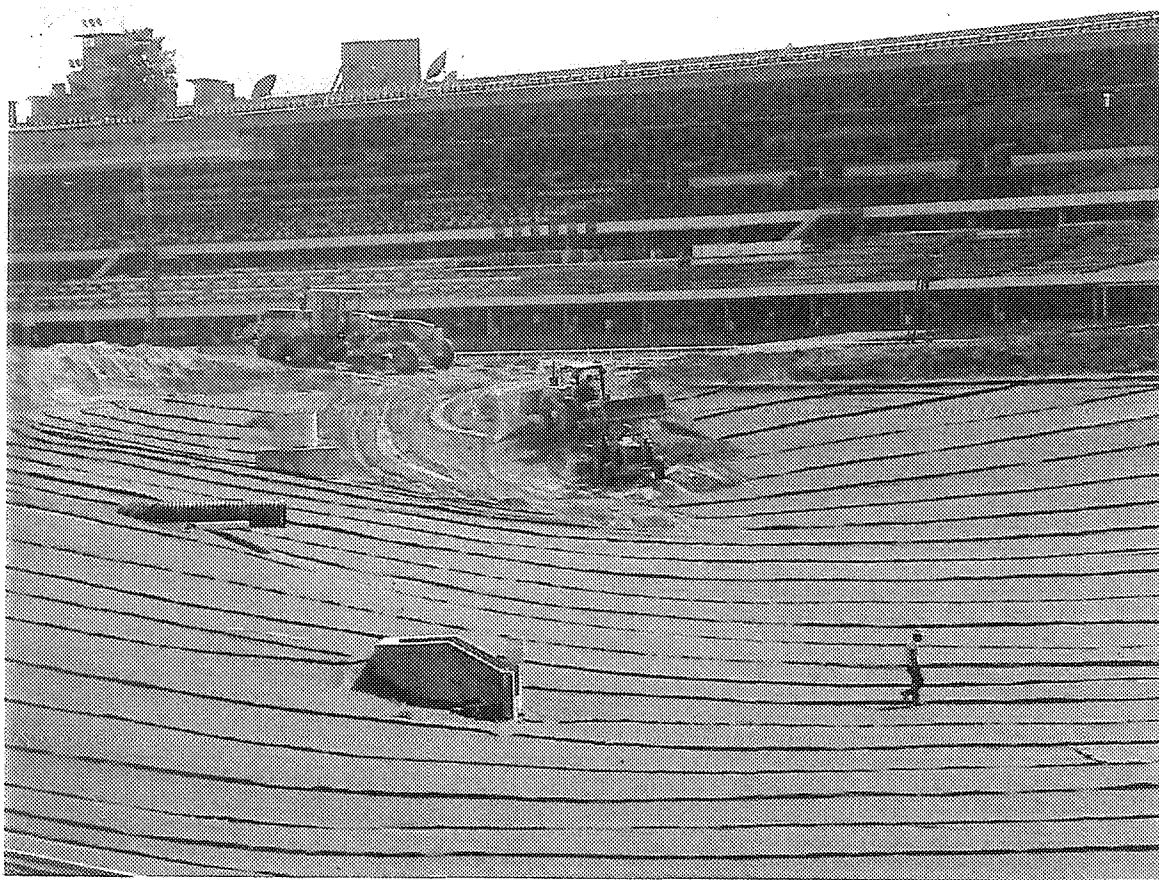
Placement of 24 inch misc. soil cover over the geotextile lining on 9/7/00.
