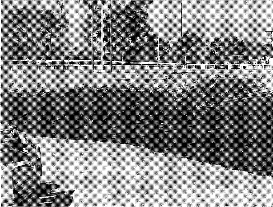
. Placement of soil cover over geotextile fabric on 9/8/00.
