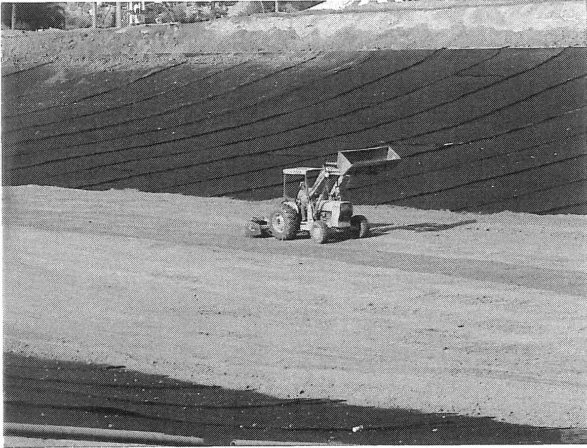
Placement of 24 inch soil cover over geotextile fabric on 9/8/00.
