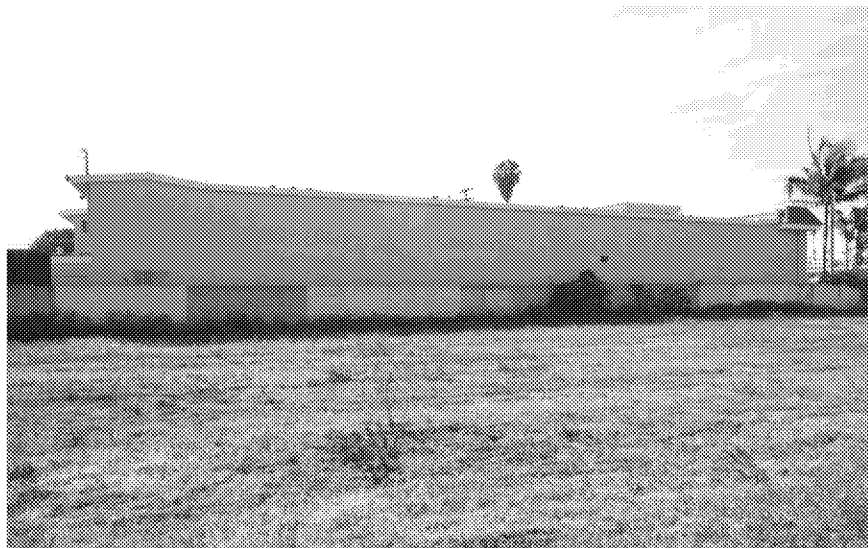
East (side) façade, view facing west. ESA, 2018.
