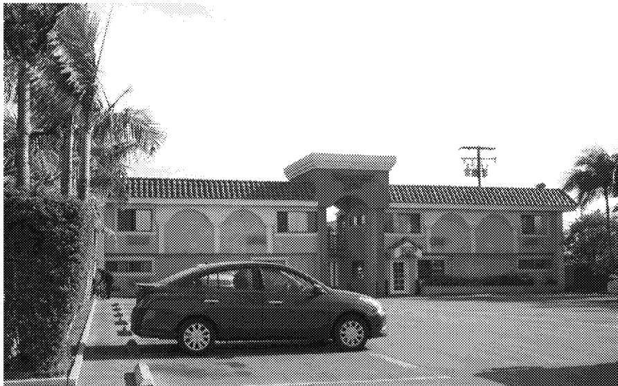
Figure 22 North (front) façade, view facing south
