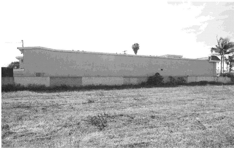
Figure 24 East (side) façade, view facing west
